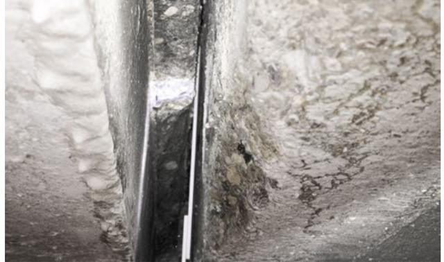
Fig. 2: Clearing joint, cleaning joint edges, cutting open joints if necessary
