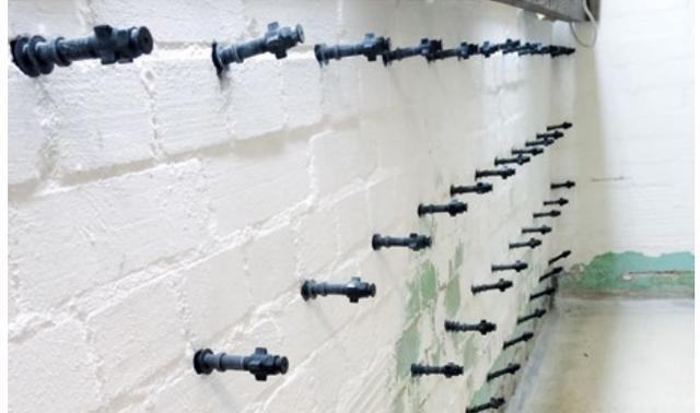
Fig. 2: Example of packer positioning
