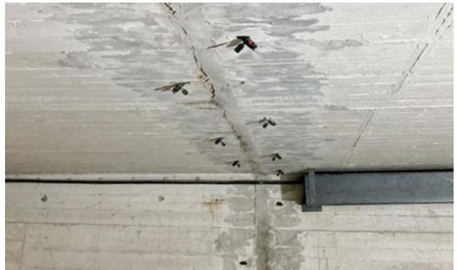
Fig. 4: Patching joint areas, drilling holes and installing packers
