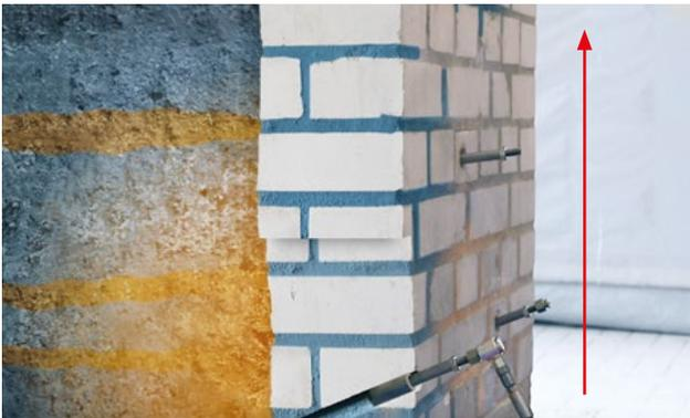
Fig. 3: Injection from bottom to top
