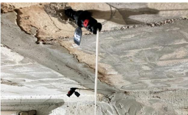
Fig. 5: Injecting material
