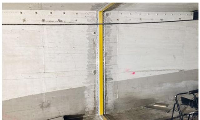
Fig. 6: Reworking joint
