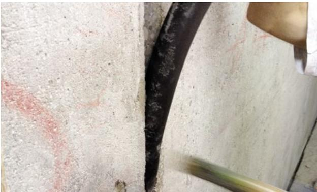
Fig. 3: Installing hammer-in profile
