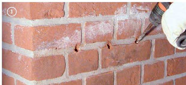
*Making of drill holes (masonry size 24 cm)*
