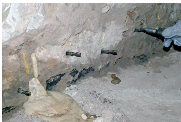
*Preliminary injection of a PU injection foam resin into masonry with cavities*
