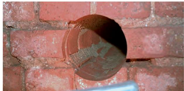
*Core removal from brickwork*
