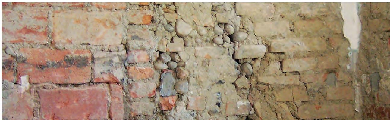
Damages in mixed masonry
