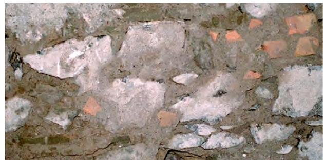
*Natural brickwork with loam mortar joints*
