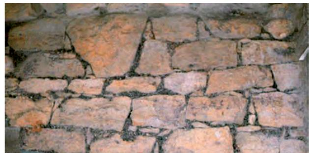
*Large-format cyclopic brickwork with large-pored joints*
