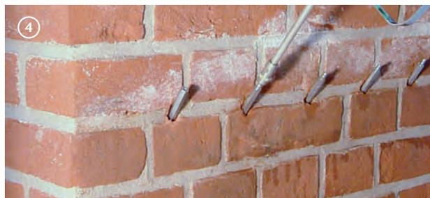
*Injection of PU injection resin*
