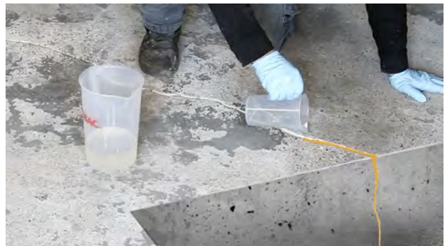
Fig. 4: Crack impregnation with epoxy resin
