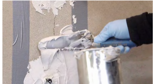
Fig. 4: Patching and gluing of the surface packers
