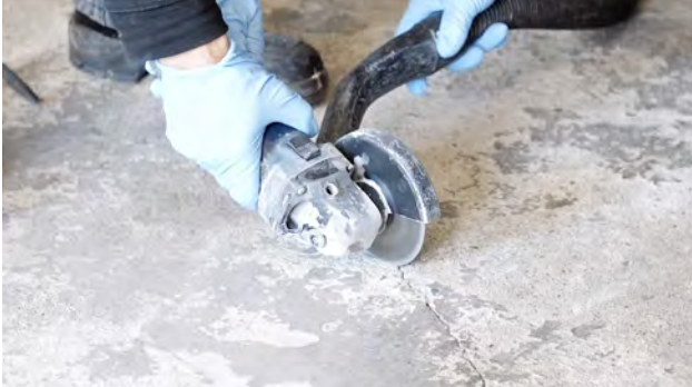
Fig. 1: Widen crack by recutting
