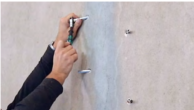
Fig. 3: Installation of packers
