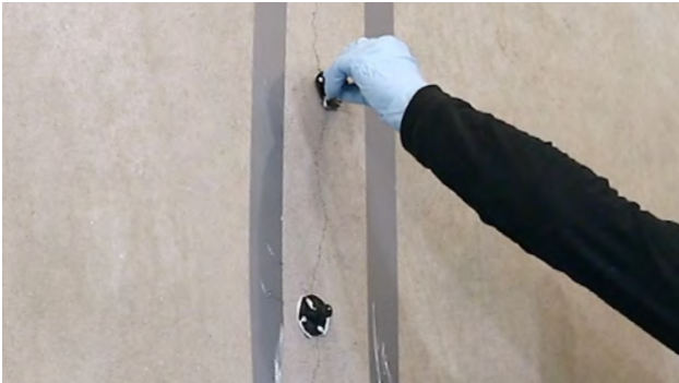
Fig. 3: Placing of surface packers
