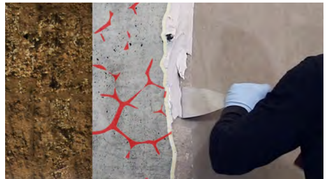
Fig. 6: Removing the patching and packers
