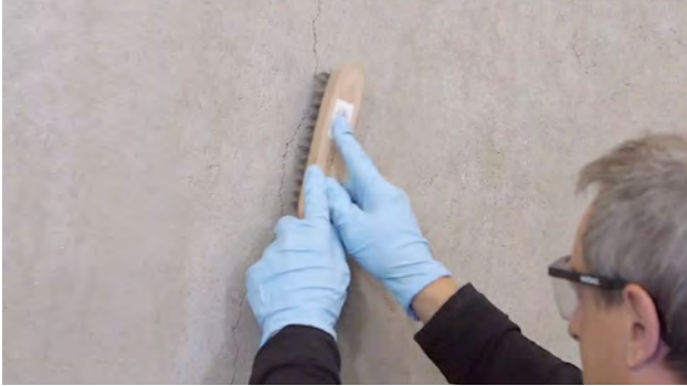
Fig. 1: Cleaning of the surface
