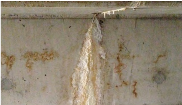
Chalk efflorescence
