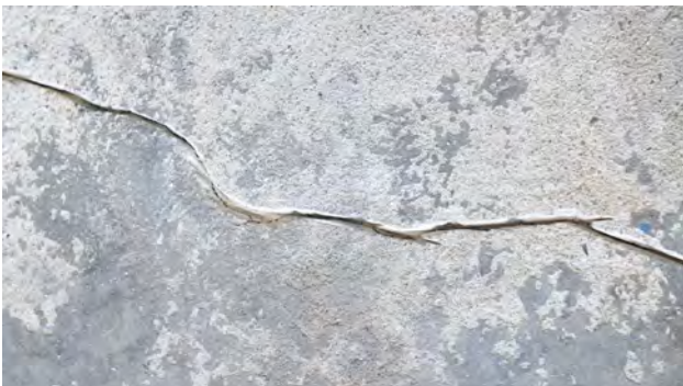
Fig. 3: Prepared crack before impregnation
