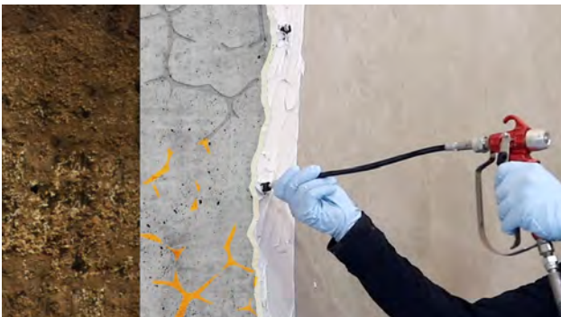
Fig. 5: Injection from bottom to top
