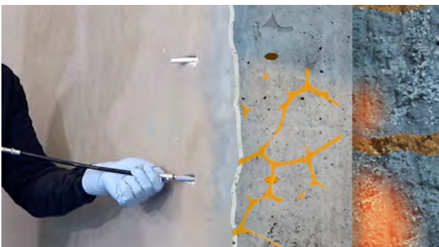
Fig. 5: Injection from bottom to top
