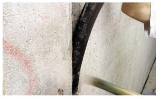
Fig. 3: Installing hammer-in profile
