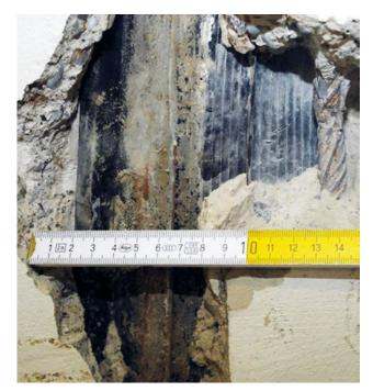
Measurement of a brittle expansion joint
