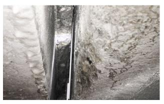
Fig. 2: Clearing joint, cleaning joint edges, cutting open joints if necessary
