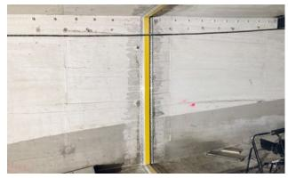
Fig. 6: Reworking joint
