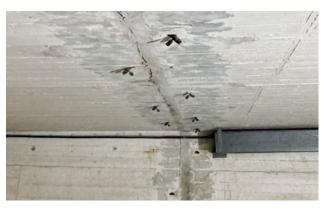
Fig. 4: Patching joint areas, drilling holes and installing packers
