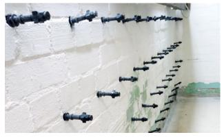
Fig. 2: Example of packer positioning
